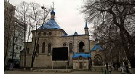
St. Teodora de la Sihla Church in Central Chişinău was one of the churches that were "converted into museums of atheism", under the doctrine of Marxist–Leninist atheism . [32]
