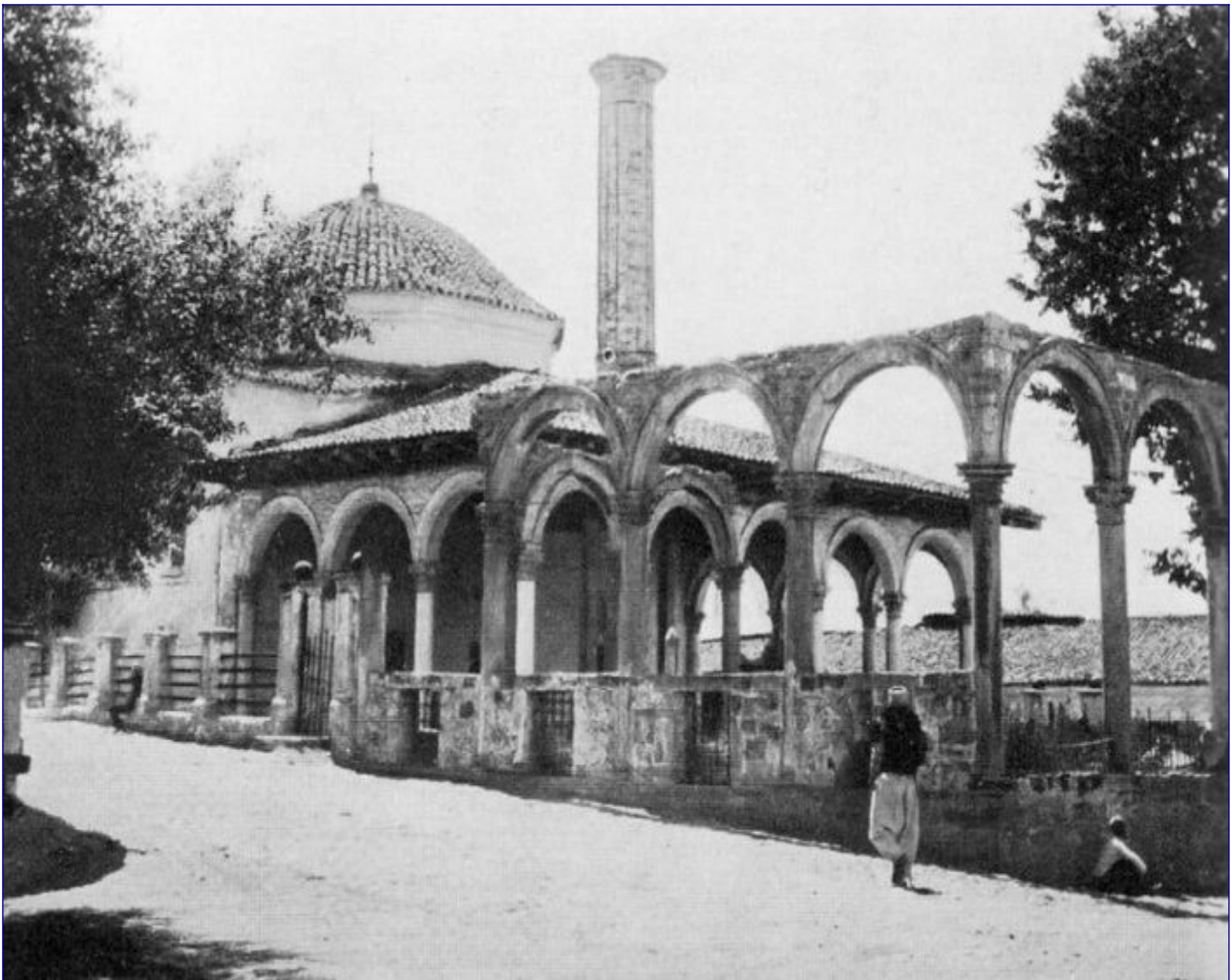
Kubelie Mosque in Albania, prior to demolition. Photo via the public domain.
