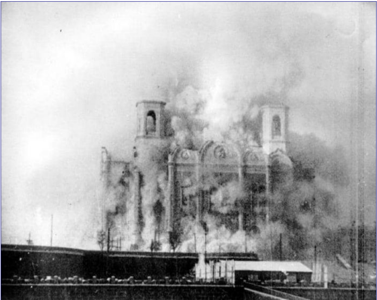
Demolition of Christ the Savior Cathedral, Moscow, 1931. Photo via public domain.
